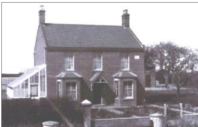
The original building before alterations (Womack View)
