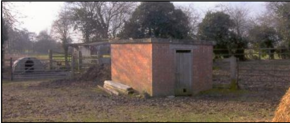
Ammunition store in Norwich Road
