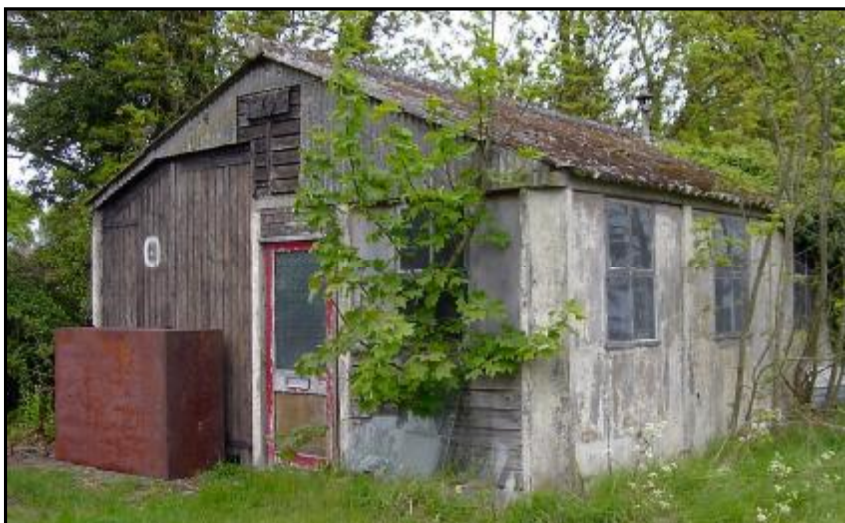
The old fire station prior to refurbishment as offices in 2006/7
