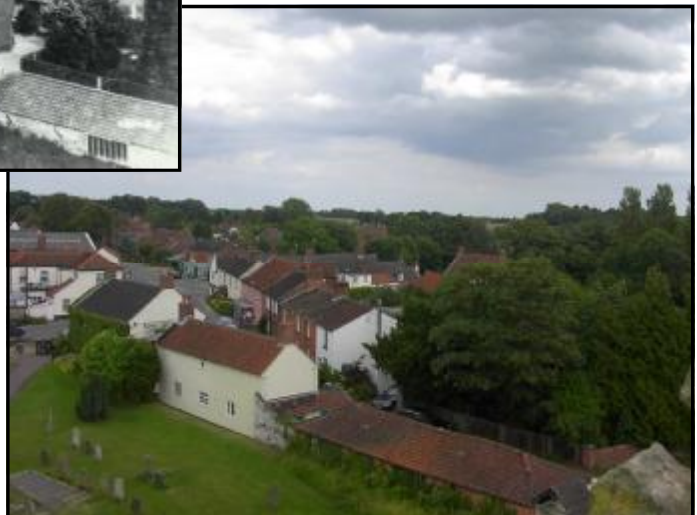
A similar view taken in June 2004 during church roof repairs.
