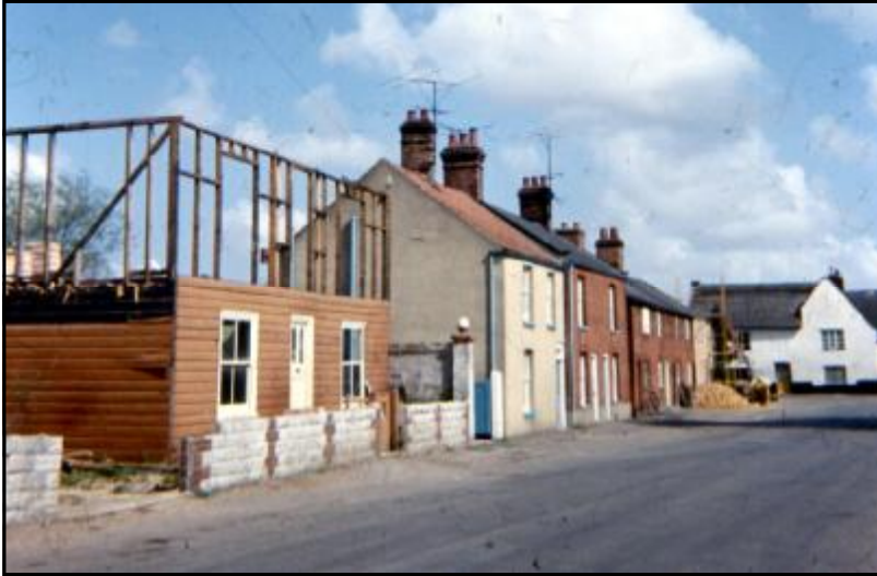
Demolishing the wooden house, late 1960's
